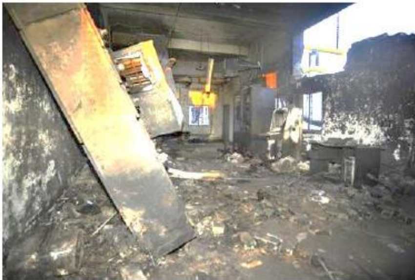
Destroyed Control Room
